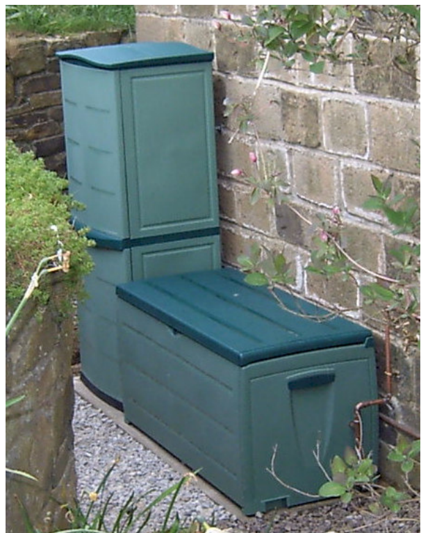
The picture above shows a SpringBox containing a household filtration system. The picture below shows the PumpBox where a booster pump is fitted inside the weather proof cabinet.
